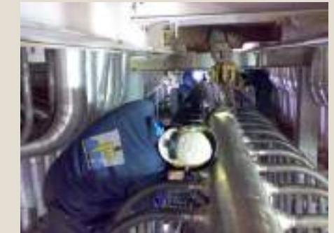
Revamp of Hydrogen Steam Reformer Heaters
