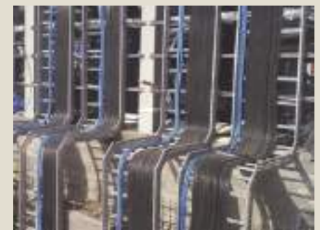
Installation of Instrument Cables
