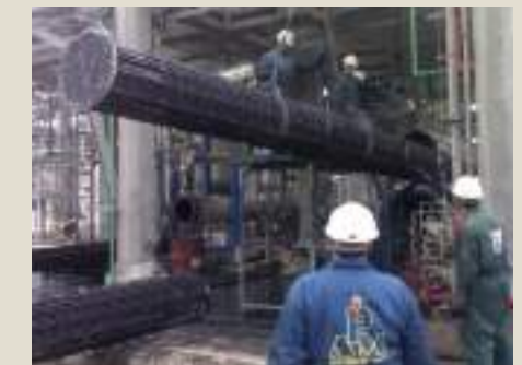
Maint. of Heat Exchangers
