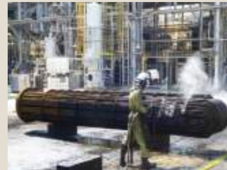
Maintenance of Heat Exchangers - SIDPEC
