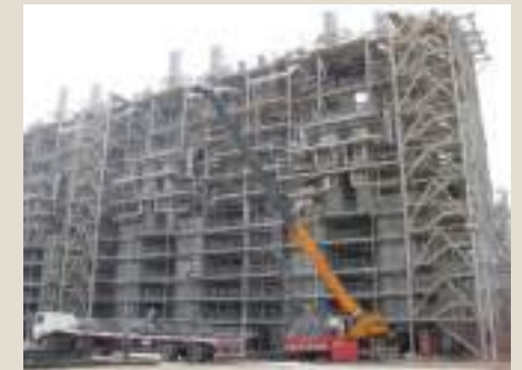
Maintenance of Ethylene Furnace - SIDPEC
