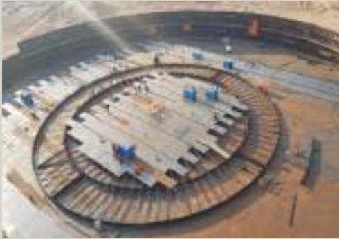
Installation & welding of tank at crude oil storage area (Ras Ghareb)
