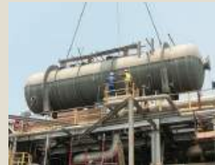
Deaerator of boiler – MIDOR Shutdown
